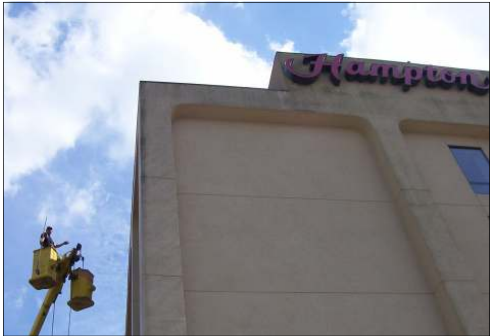
ECO-FIRST employee Sterling Ayers pressure cleans a Hampton Inn hotel atop a 100-foot bucket truck. ECO-FIRST specializes in industrial and commercial cleaning. Photo by ECO-FIRST, Inc.
